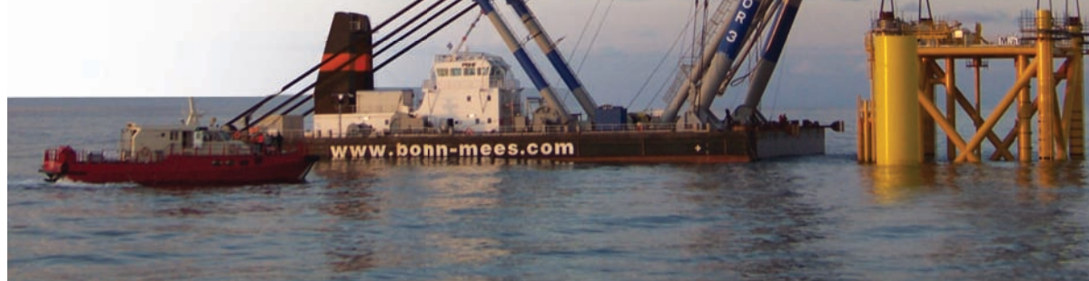
Matador 3 in action on open-water construction site
